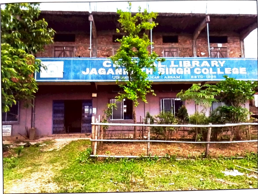
Front view of Library Building
